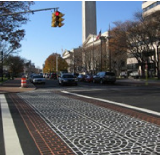
Crosswalks and traffic calming devices at street corners can be as simple as thermoplastic markings that visually identify a pedestrian zone or as detailed as special brick or granite pavers.
