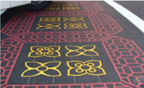
Custom shapes can be manufactured for crosswalk designs. Goldfish, artesian wells and Old Hickory emblems have been mentioned in public meetings. Thermoplastic embedded and integrally colored heat applied finishes are available for long lasting color.
