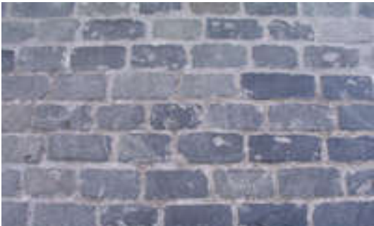
Brick pavers, a long tradition for Martinsville street surfaces, could be inlaid for crosswalks. However, repaving of the streets in the future is problematic with this type of installation.
