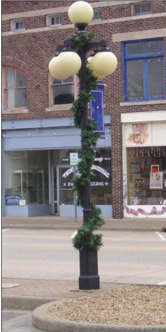
Existing light pole attempts to capture the historic quality of poles that were used in the early part of the 20 th century. There have been problems in maintaining the 5 globes per pole and non-working globes give a general feeling of neglect even though lights are maintained on a regular basis.
