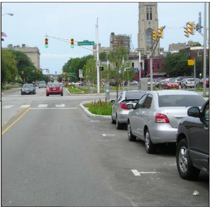
Above and below are examples of traffic calming islands at street corners. The islands pictured are a part of the Indianapolis Cultural Trail which uses the islands not only for pedestrian and bicycle safety but also for storm water quality. Each island contains native perennials that help clean storm water that drains into the sunken rain gardens from adjacent streets.
