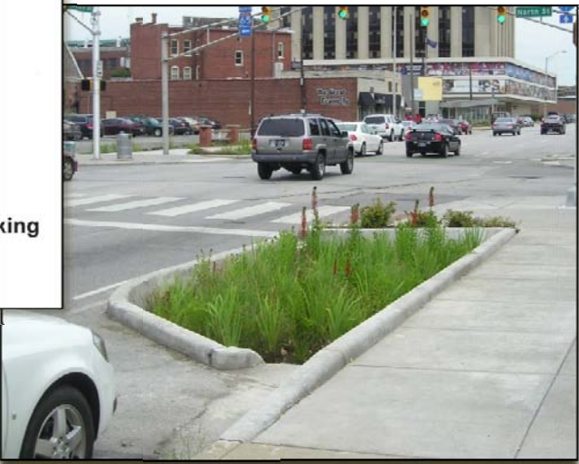
Above and below are examples of traffic calming islands at street corners. The islands pictured are a part of the Indianapolis Cultural Trail which uses the islands not only for pedestrian and bicycle safety but also for storm water quality. Each island contains native perennials that help clean storm water that drains into the sunken rain gardens from adjacent streets.
