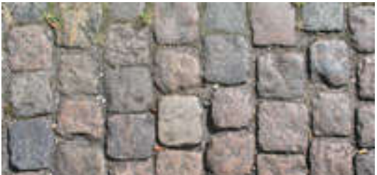
Stone pavers provide tactile warning for cars entering pedestrian spaces but are difficult to walk on.
