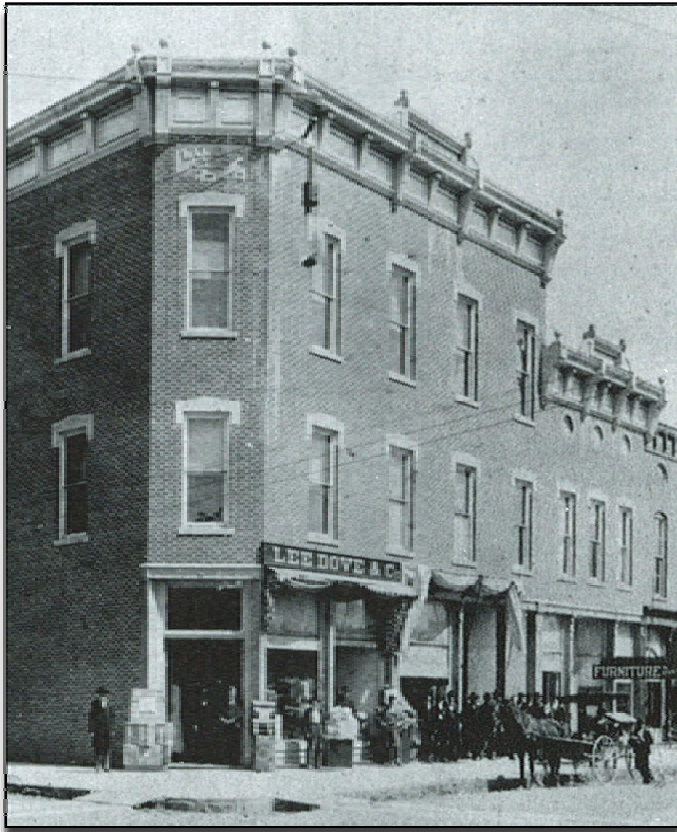
The original Independent Order of Odd Fellows (I.O.O.F.) building photo c.1895 shows large storefront windows with clear glass transom windows. Note that the entrance door currently inset, was set flush with the corner face of the building.
