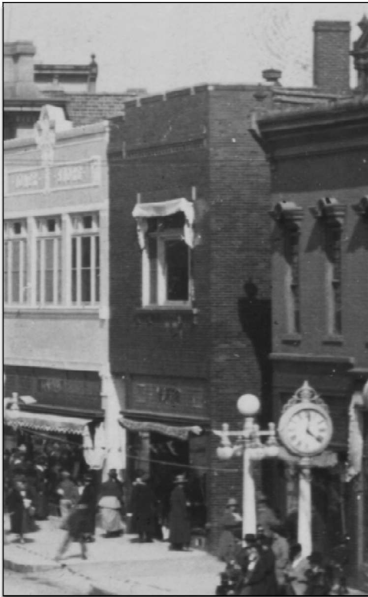
This c. 1922 photo shows that the upper window layout of the building has changed but the brick surround has remained intact. The lower part of the building is indicative of other commercial store fronts of the time with small pane textured glass transom and large clear storefront windows. Note ornamental street clock in foreground.
