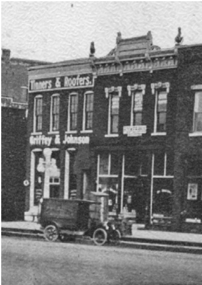
This c. 1916 photo shows that the façade on 29 East Washington has been significantly changed. Brick columns separated the 3 bays of the façade. These brick columns have been removed but the larger storefront windows and open transoms are still in keeping with the age and scale of the building, so new brick columns have not been proposed.
