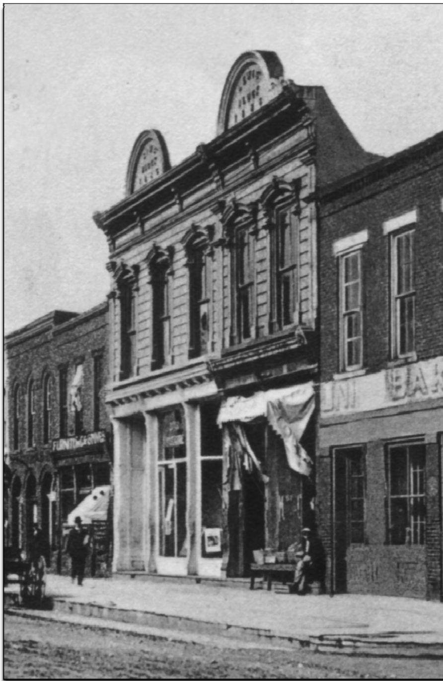
This c. 1910 photo of 78 East Morgan shows rounded architectural elements along the top parapet walls which are no longer in place. This proposal does not replace those elements due to lack of architectural details and anticipated cost to reproduce.
