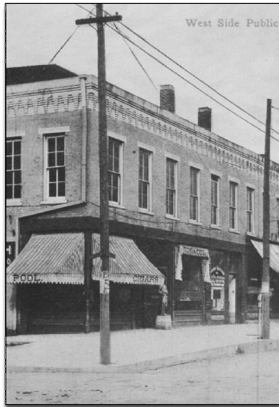
These c.1910 & 1904 photos show the prominent cornice that separates the brick façade from the lower storefront windows and transoms. Wood bulkheads below the storefront windows can also be seen below the awnings.
