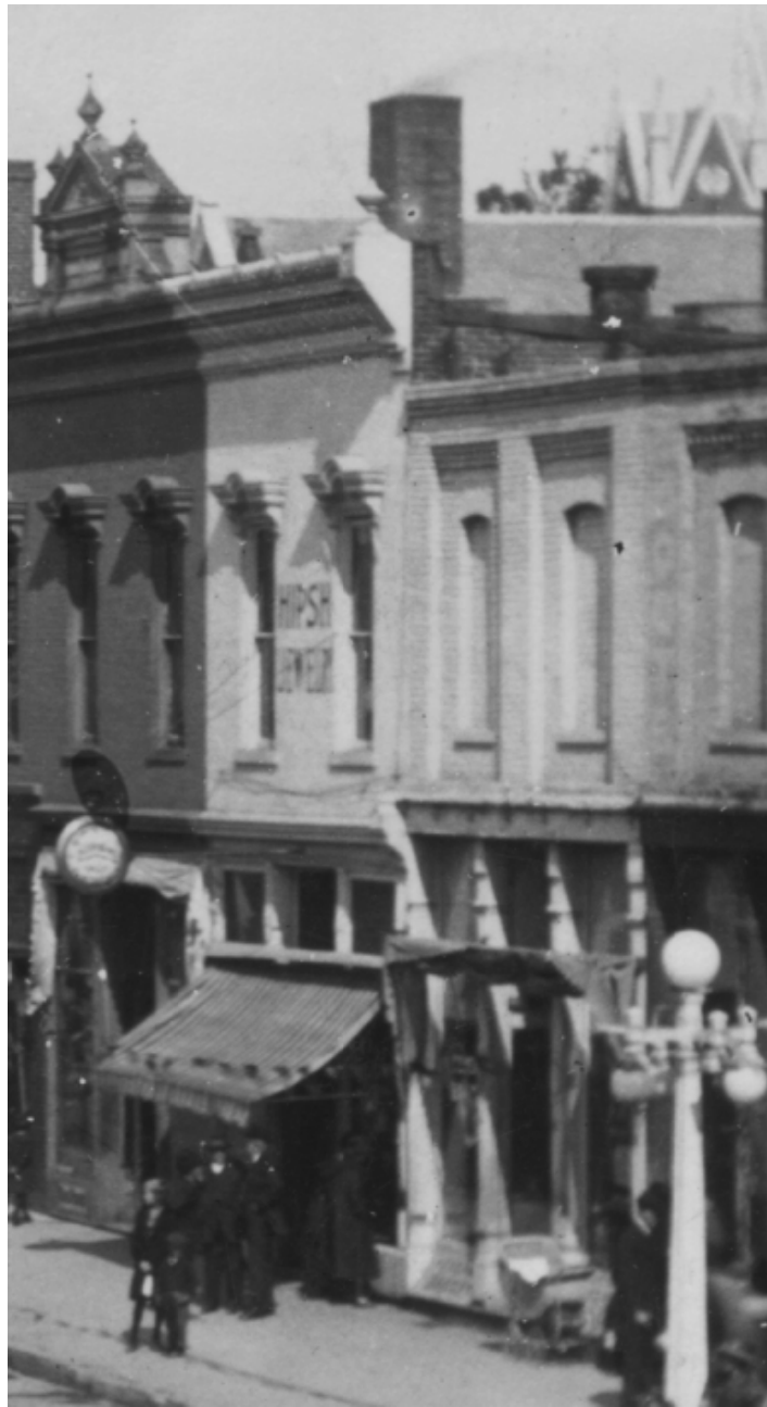
This c. 1922 photo shows that the upper level of 27 North Jefferson, the building to the right of Hipsh Jewelry, has been significantly altered and the upper windows removed. While it might be nice to recreate the upper windows, the current upper building façade retains some historic precedent of its own and should not be changed.
