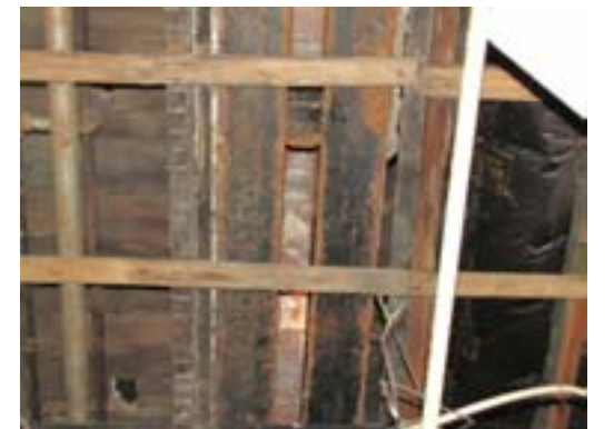
P10 - Bottom of the double steel beam supporting the upper masonry wall at the rear of the two story wing.
