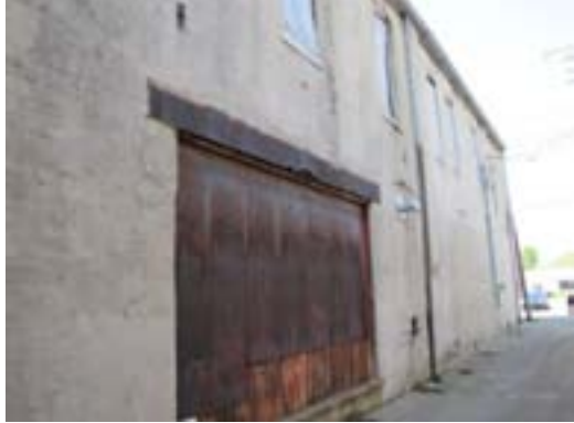
P2 - Opening on the north side of the building. This opening should be filled with new concrete block. Note the corroded lintel.
