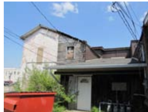
P13 – View of the rear of the building. Note the deterioration of the wood framed portion of the west wing addition.
