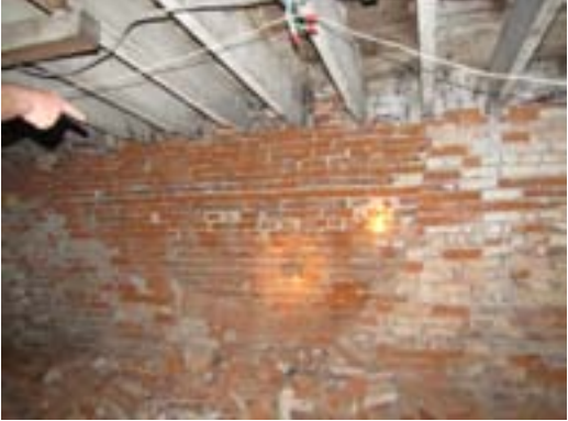
P4 - Collapsed brick in the basement. Joist end bearing is compromised by this collapse.
