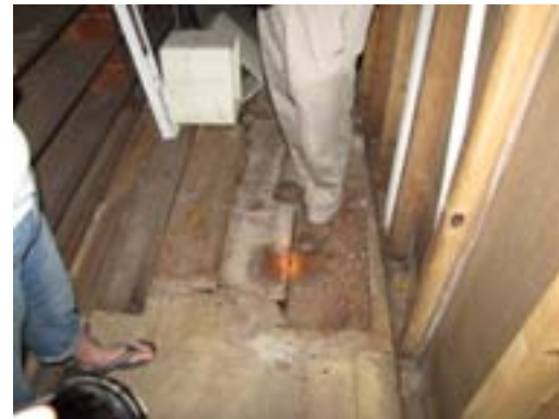
P12 - Spongy and sagging floor area at the south side of the first floor.
