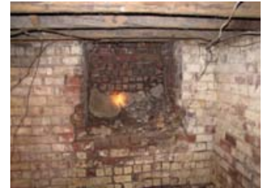
P10 – Abandoned coal chute in the south basement wall under the art store. This is one point of entry for water.
