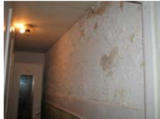
P7 – View of the inside of the east wall of the Veterans Museum. Note the peeled paint due to water leakage.
