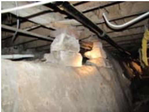
P6 - Stone and wood shim joist support on either side of the dirt basement tunnel. Note loose laid stone units.
