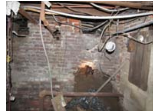
P5 – Collapsed basement wall. This occurs under the severely sagging area of the first floor.
