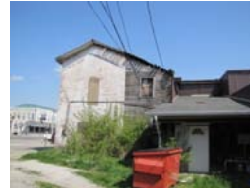
P4 – View of the rear of the building. Note the wood framed portion of the west wing addition and the one story infill addition.
