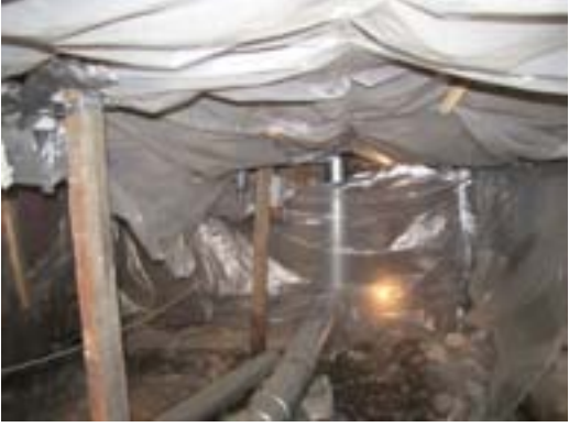
P9 - Rear compartment of the basement. Note the wood posts and beams providing additional floor joist support.
