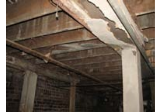
P5 – View of the first floor framing under the Veterans Museum showing wood joists and wood beam.
