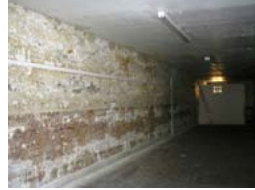
P14 – Close up view of the second floor, east wall of the building. This wall was exposed to fire in the past.
