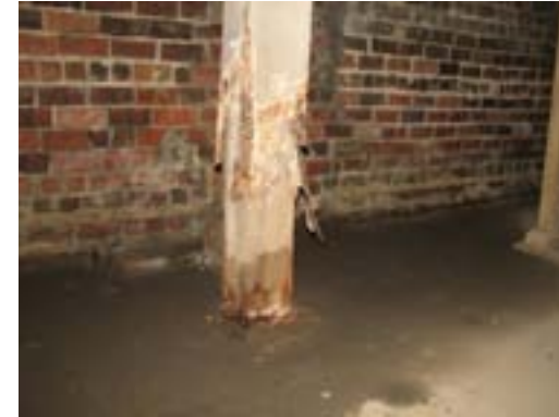
P4 – View of the base of a wood post under the first floor of the Veterans Museum. Note the water damage.
