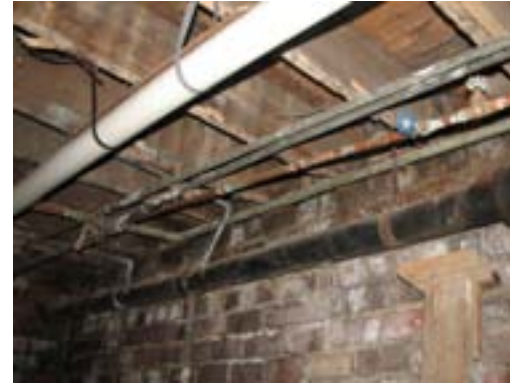
P3 – View of water damaged joists along the east side of the Veterans Museum first floor.
