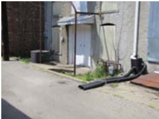
P6 – Close-up of the rear of the building. Note the low grade against the building.
