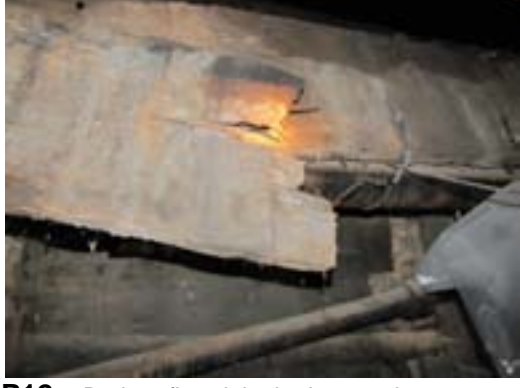
P12 - Broken floor joist in the rear basement compartment.
