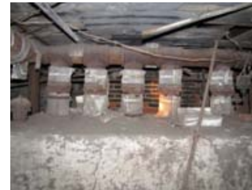
P14 – View of the abandoned boiler in the basement. May represent a hazardous material condition.
