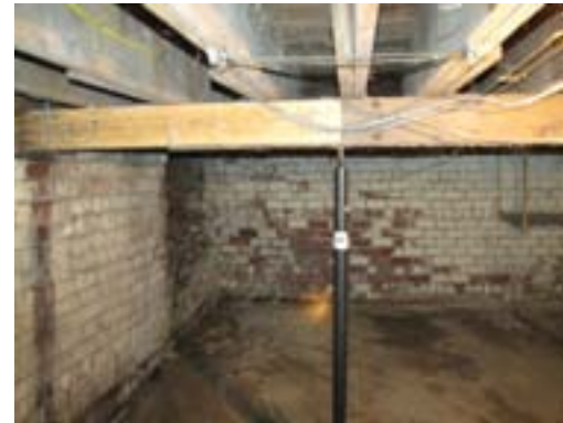
P8 – View of beam repairs and a new steel jack column in the basement under the art store.
