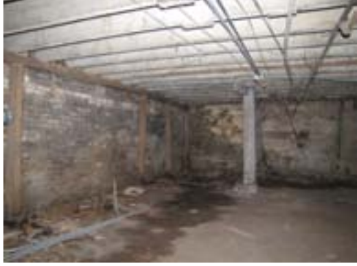
P7 - View of the front compartment of the basement. Note the wood posts and beams providing additional floor joist support.
