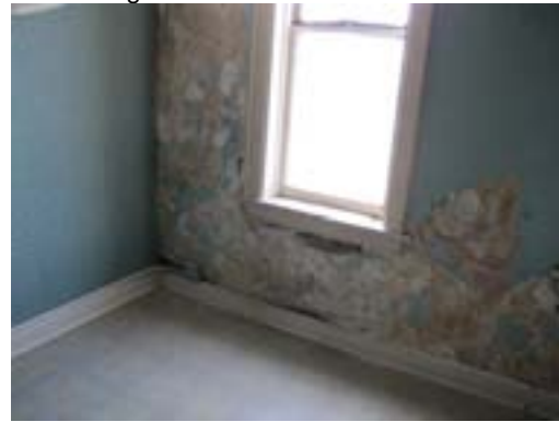
P8 - Upper level exterior masonry wall at the rear of the two story wing. Note the water damage to the inside face of the wall.
