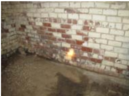
P11 – View of the basement wall under the art store looking southwest. Note the water damage to mortar joints.
