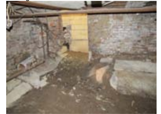
P15 – View of the basement looking south. Note the crumbling concrete at the base of the wall and the wet dirt floor.
