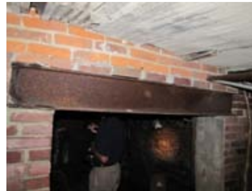
P8 – Corroded steel lintel over a basement wall opening.
