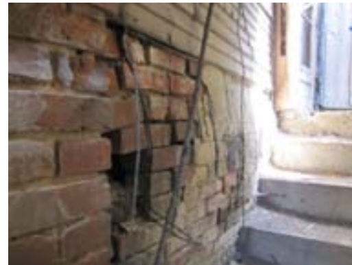
P7 – Partially collapsed and bowing brick masonry on the north side of the rear stair that leads to the basement.
