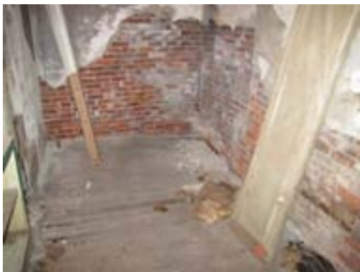
P11 - Spongy and sagging floor area at the south side of the first floor.
