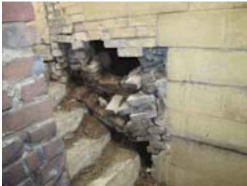
P6 – Partially collapsed block masonry on the south side of the rear stair that leads to the basement.
