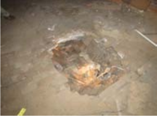
P5 - Collapsed cistern in the basement within the front compartment.
