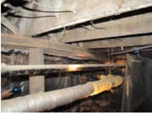
P8 - Rear compartment of the basement. Note the wood posts and beams providing additional floor joist support.
