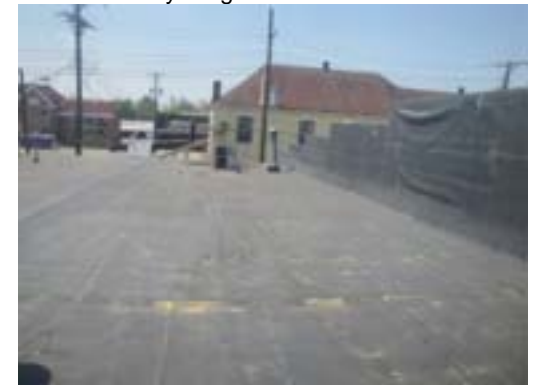
P15 - View of the roof over the one story wing looking west. Rubber membrane roofing.
